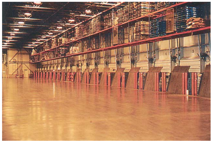
The dock area features Serco vertical dock levelers. Overhead storage space is provided for empty pallets above the 24 door locations. Up to 2300 pallets can be stored in this fashion.
